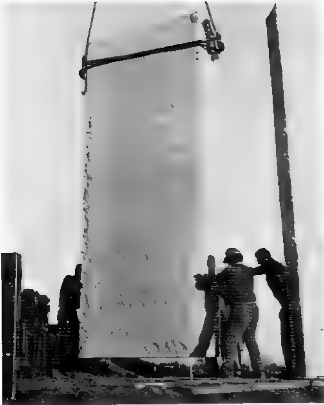
“Ever so gently!” describes how the crane and setting crew handled the stone sections and their enormous weight. As shown above, stainless steel dowel pins were placed in each of the granite bases and the upright sections were set on the pins.
